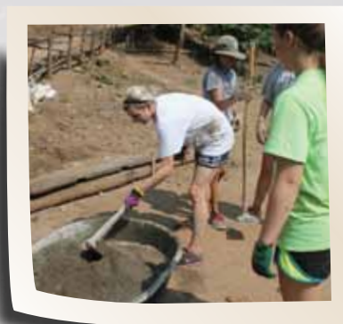
Ashley building the water tank foundation.
